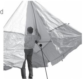
9. Align the bottom rods on the right side so that they are in the correct position and at an appropriate distance apart and then stretch the tent wall taut by pressing the fixation disc (B) towards the outer tent wall until the side frame is under tension
